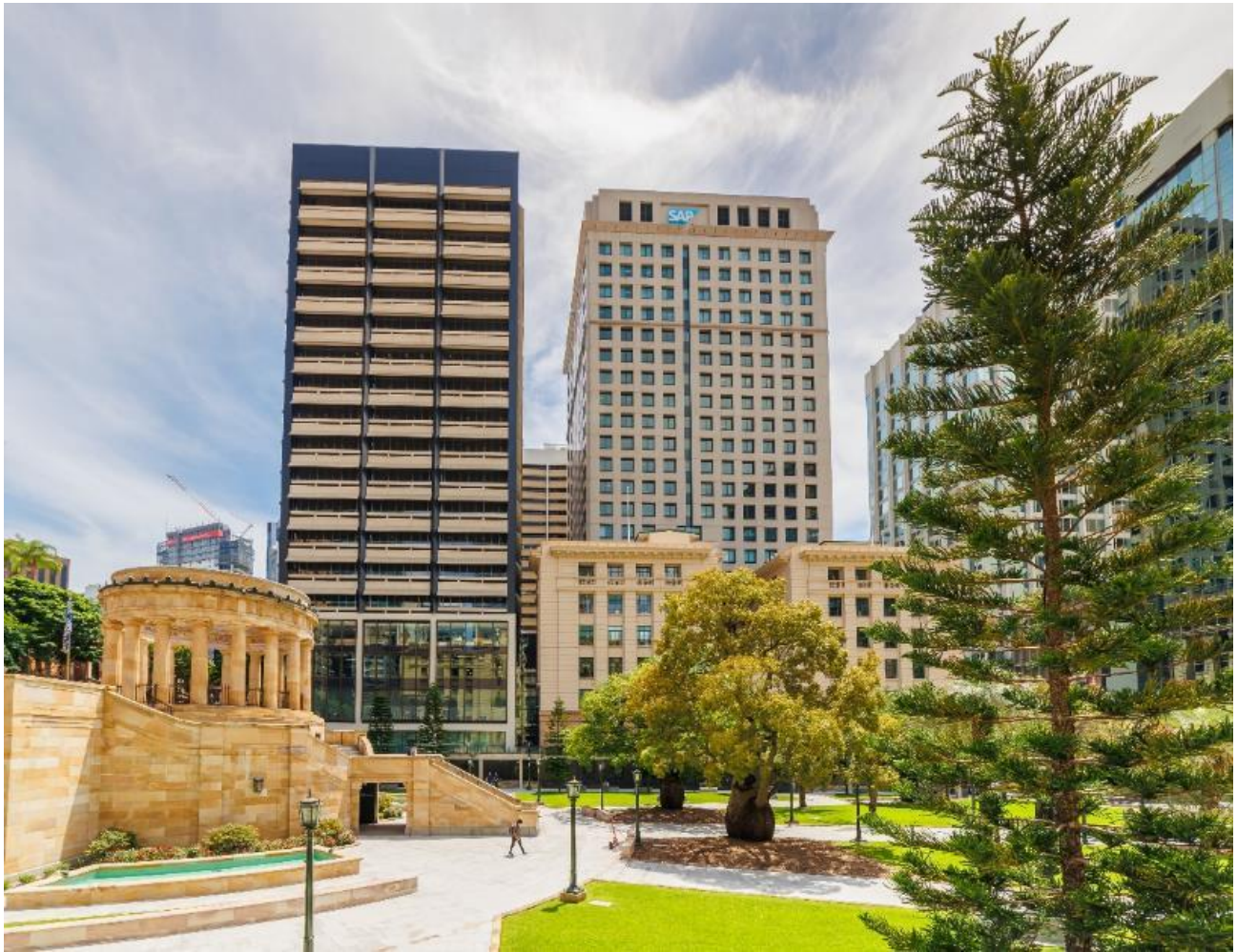
External shot of No1 ANZAC Square showing new façade to 295 Ann Street
